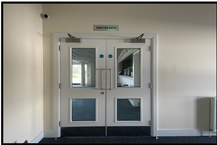
Entrance doors to the Function Suite
