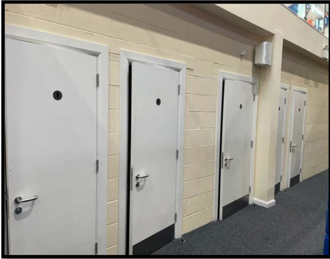
Activity Centre toilets (Play Frame side)
